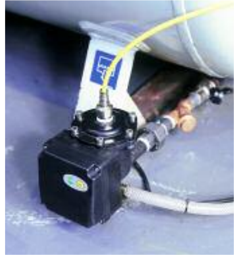
ED2100 installed on a compressor/receiver package.
