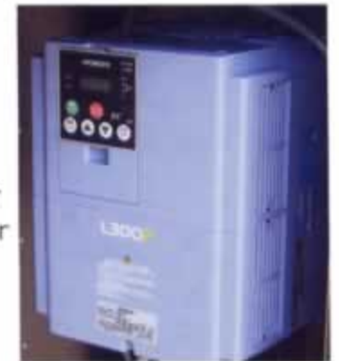
frequency enhanced inverter
